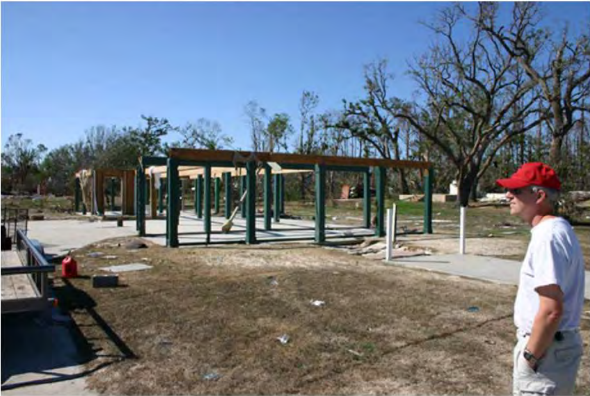
Remains of Rear Admiral Dave Titley's house after a nine-meter storm surge on the Gulf of Mexico
