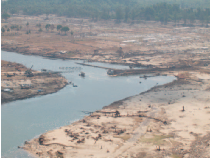
Destroyed bridge, cutting north-south road traffic, Aceh Province.
