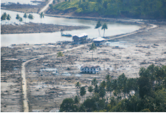
Tsunami damage at Pasi, northwest coastline of Aceh Province.
