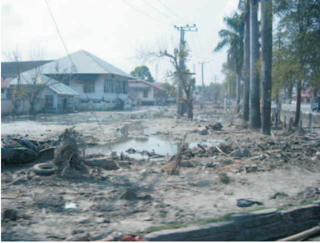
Extensive urban destruction, Aceh Province.
