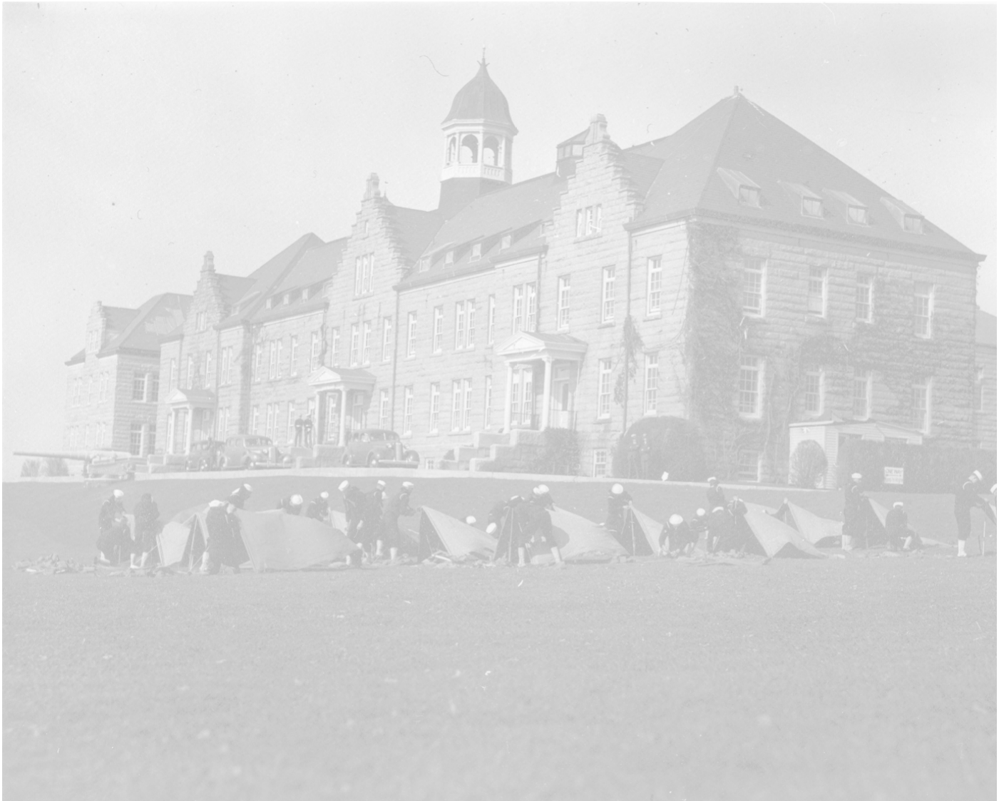
Luce Hall, c. 1938. Recruits of the Naval Training Station (housed in what is now Sims Hall) are pitching tents on Dewey Field.
