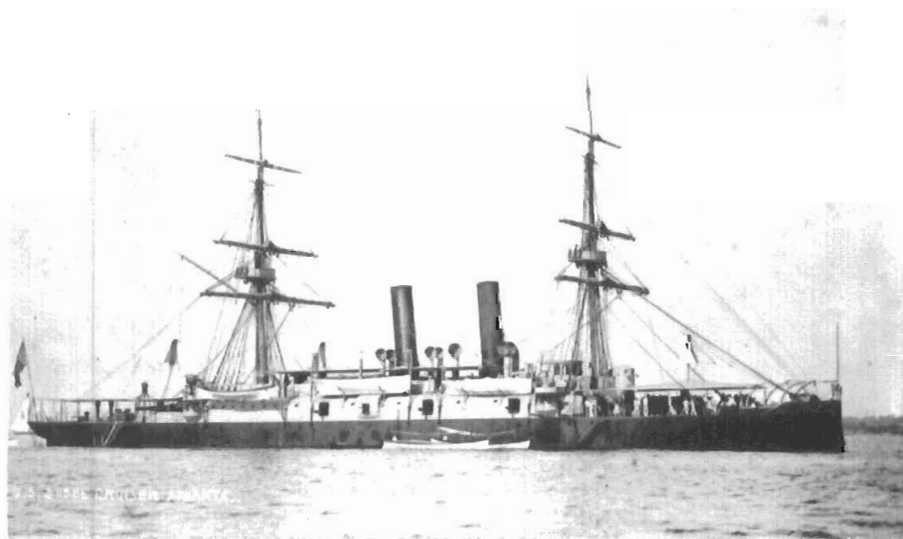
Luce's most powerful ship, the steel protected cruiser Atlanta . She and the dispatch boat Dolphin were the first ships of the "New Navy" begun in 1883. Commissioned in 1886, the Atlanta displaced 3,189 tons. She was armed with two 8-inch, six 6-inch, and a number of smaller weapons. Her speed was 15 knots.
